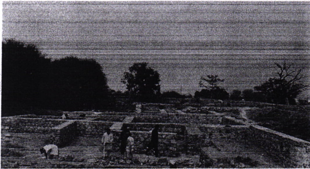
Fig.10: General view showing ongoing conservation work at Sirkap
