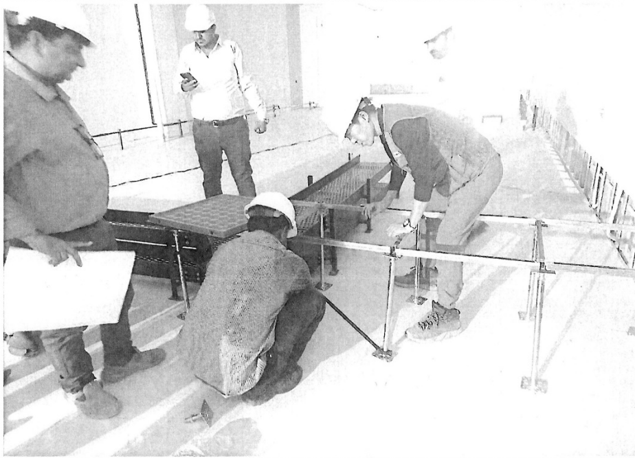
Raised Floor Pedestals Installation
