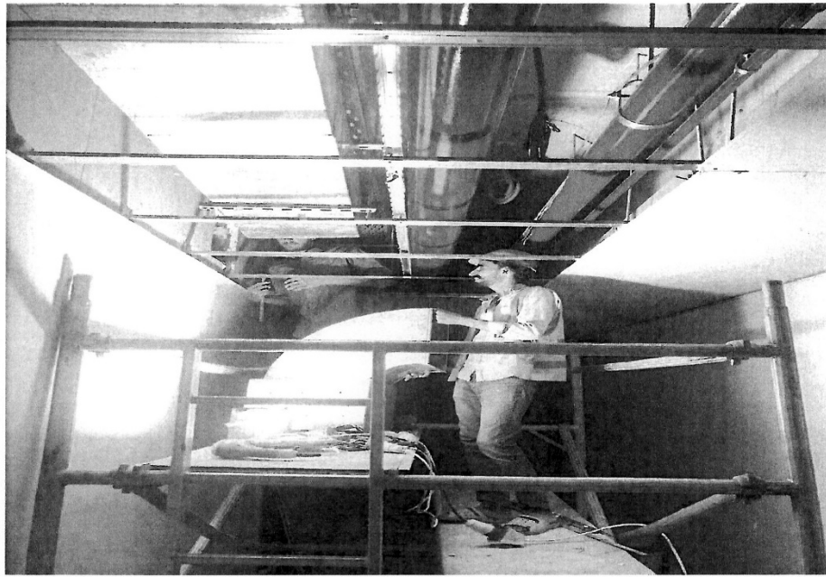
Fire Fighting Piping Works
